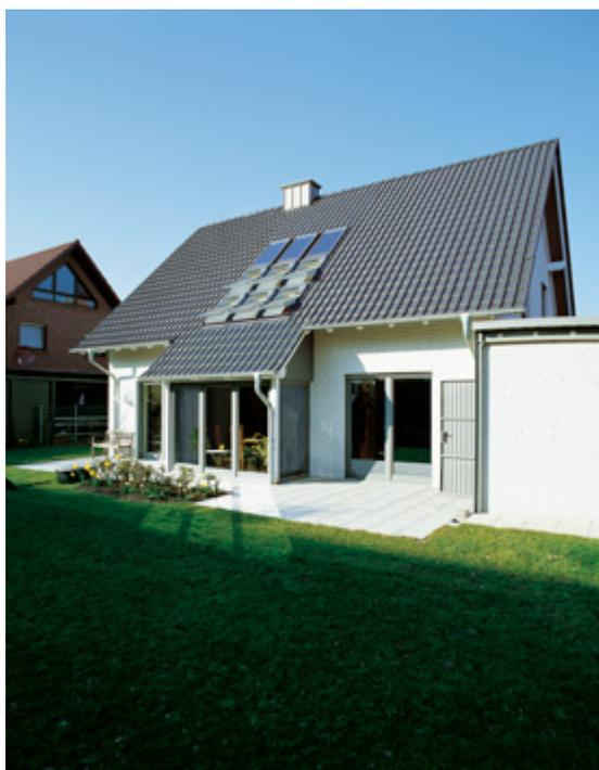
Skylights are light transmitting fenestration that form all, or a portion of, the roof of a building space. Skylights can either be in the form of roof windows, unit skylights, tubular day-lighting devices
